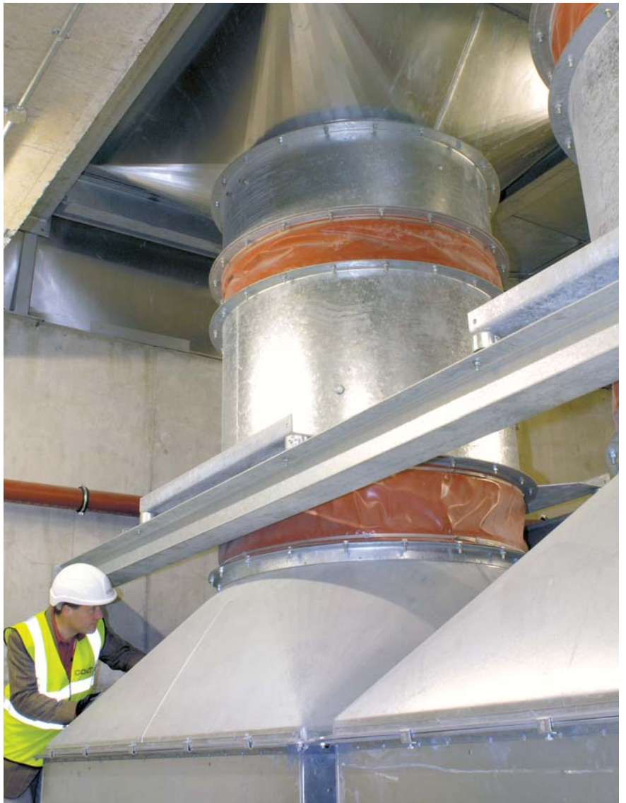
Extract plant at Gunwharf Quays, Portsmouth
