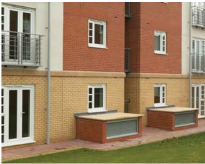
Louvre terminations at the Observatory Apartments, Walsall
