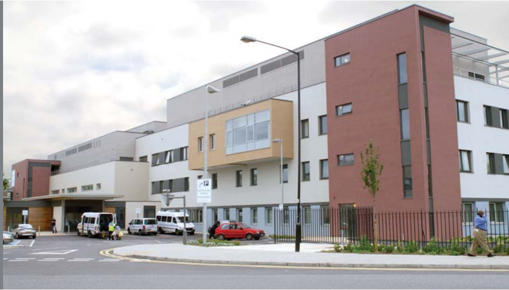
Becad Hospital, Middlesex By re-assessing the design, Colt was able to reduce a competitor's 35 impulse fans to 12 Cyclone induction fans.
