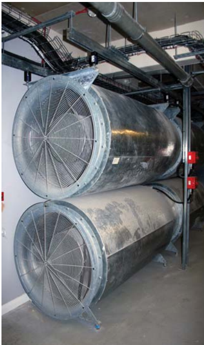
Extract fans at The Foundation, Liverpool
