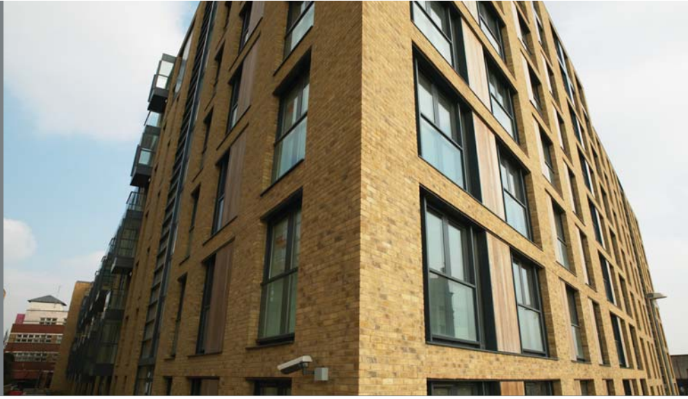
B5 Southside, Birmingham 2 Inlet Fans, 13 Cyclones, 2 Extract Fans, Dampers and Grilles, CO & Smoke Detectors
