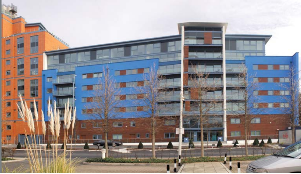
East Side Plaza, Gunwharf Quays, Portsmouth 8 Cyclone induction fans and 3 Jetstream impulse fans move the air from the entrance ramp towards the extract system, which was also supplied by Colt.
