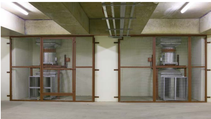
Extract plant at the Observatory Apartments, Walsall
