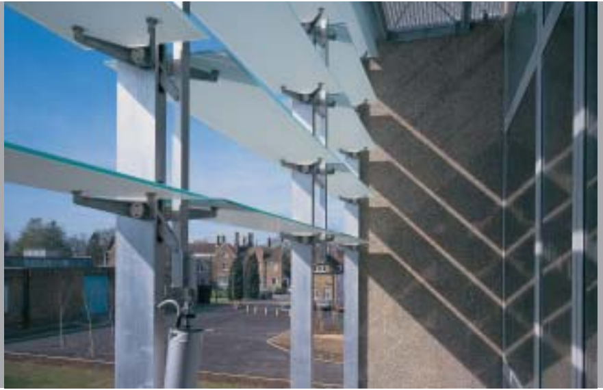
BRE Building 16, Garston, Watford.
