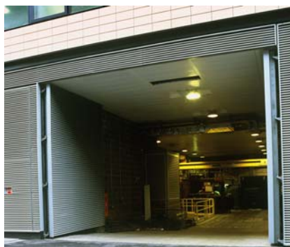
UCL, London. Louvre doors to loading bay.
