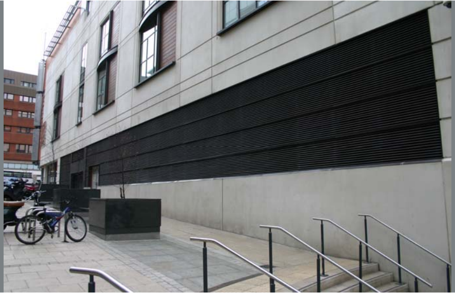
The Light, Leeds. Single bank 1UL louvre upgraded to 3UL for "live" areas.
