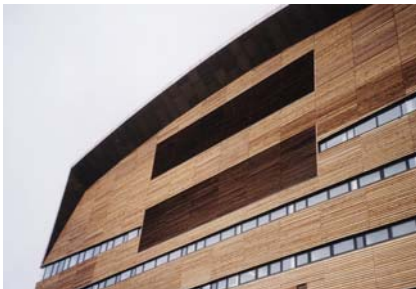
Wales Millenium Centre, Cardiff. Rough cut wooden IULIDH louvres.
