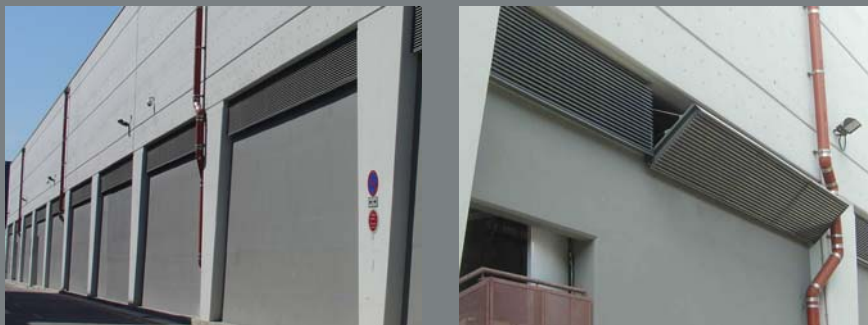
Mass Transit Railway Corporation (MTRC), Hong Kong. Side vents fitted externally with Colt Universal Louvre in line with surrounding Colt Louvre panels.
