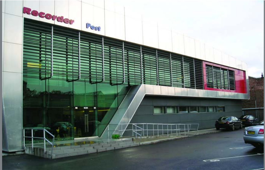
Ilford recorder, Ilford. A series of movable Solarfin louvres were integrated into a "PIA" mullion-integrated actuation system consisting of box section mullions with hidden mechanisms inside, controlled by a Colt ICS 4-Link control system.
