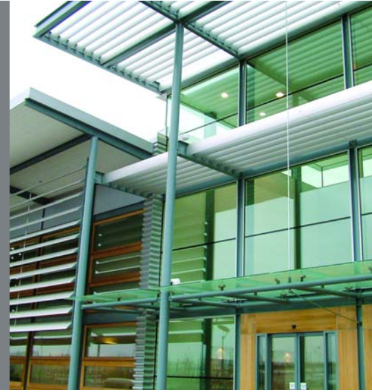
John Lewis, Cambridge. Solarfin fitted both to the customer entrance canopy and in front of the facade.
