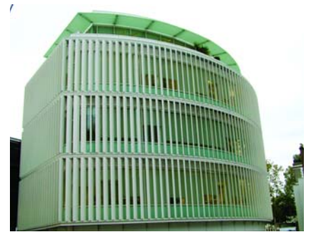
Clear Channel Outdoor, London. Both fixed and movable vertical Solarfin louvres installed onto the facade.
