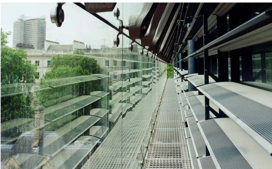
Natural History Museum, London. Between the Colt glass façade and walkway of the stunning South façade is a bespoke, controllable fin, which is half perforated to provide additional daylight when in the closed position
