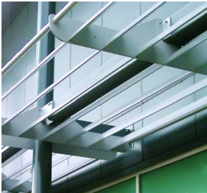
Asda, Poole. Fixed Solarfin fitted to vertical steel supports.
