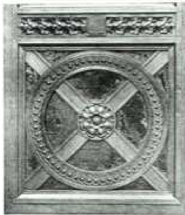
Detail of Bronze Panel showing Cast Enrichment of Doors to Main Entrance, Bedford Road
