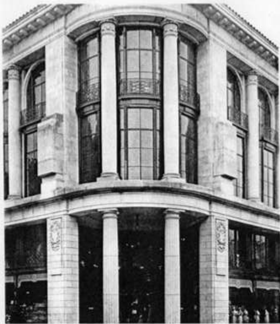
CIRCULAR CORNER: WHITELEY'S STORES Windows the same as on the front elevation, but circular on plan. Note the fire-resisting electro glass secured to the casements with solid metal glazing beads.
