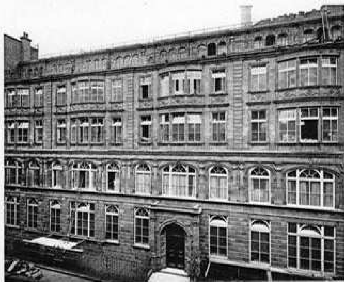
PORTION OF EXTENSION TO HARROD'S STORES, LONDON. DESIGNED BY A. W. STUBBS. Crittall steel windows with ornamental steel panelled transoms and mullions (see detail E, page 25).
