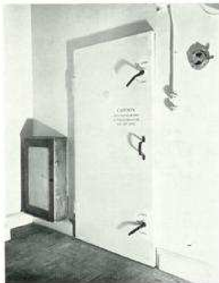
Crittall Gas-Proof Door fitted at the St. Martins Street Library, for the City of Westminster.
