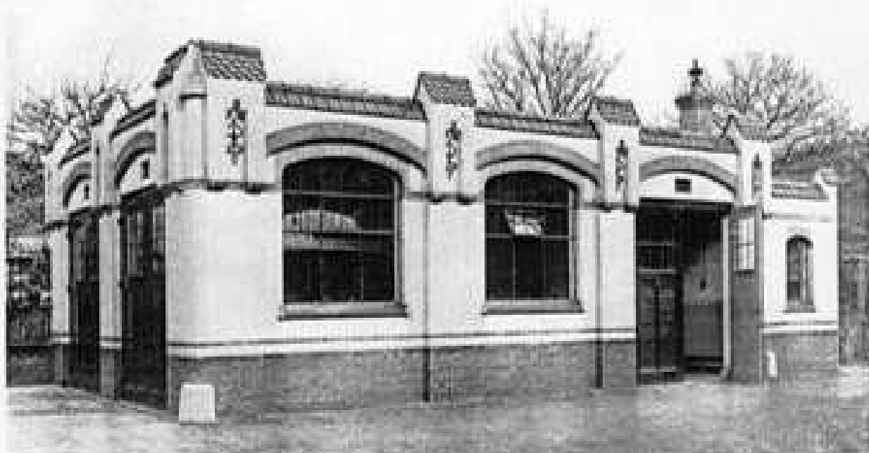
MOTOR GARAGE AT THE STABLES OF THE ROYAL PALACE, THE HAGUE, HOLLAND, FOR H.M. QUEEN WILHELMINA. DESIGNED BY SCHALTKEMA. An elegant little installation of Fenestra windows. The glazing bars in the wood doors are also Fenestra.
