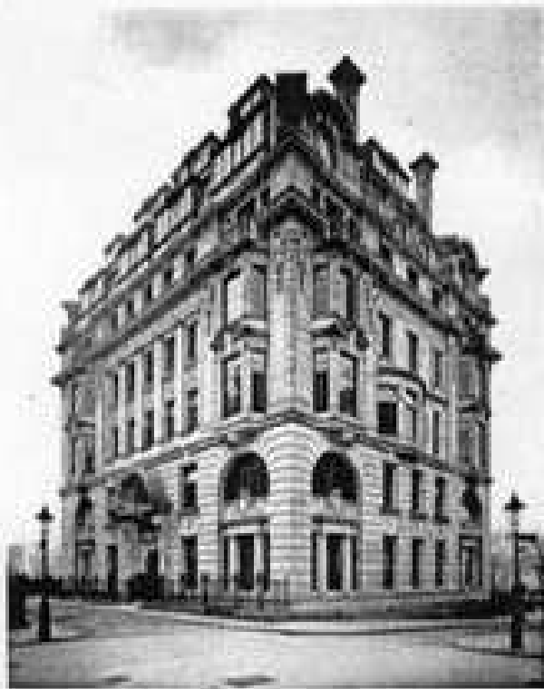
OFFICE OF THE ANGLO-AMERICAN OIL Co., WATERLOO, S.W. ARCHIT. ERNEST RÜTZE Casements divided into panes with Fenestra glazing bars.
