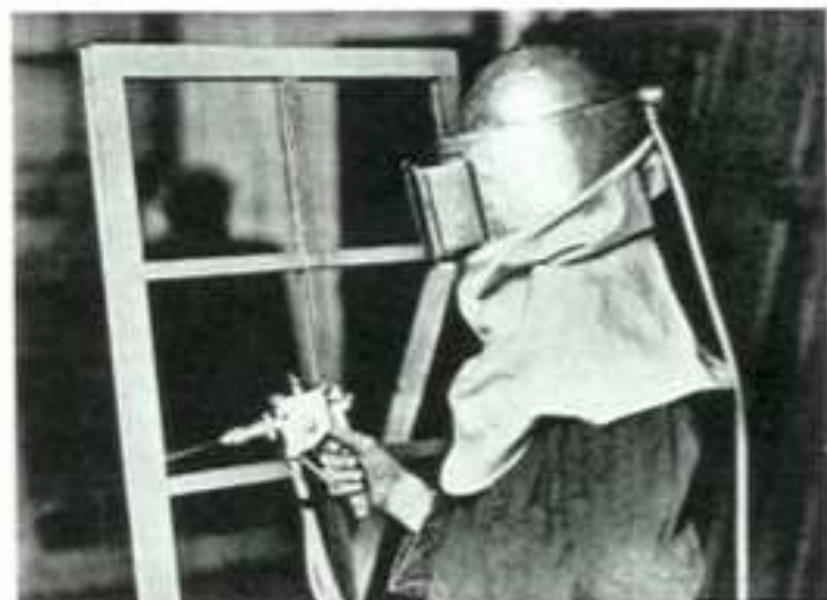
ZINC WIRE IS FED INTO A "PISTOL" AND ATOMISED
