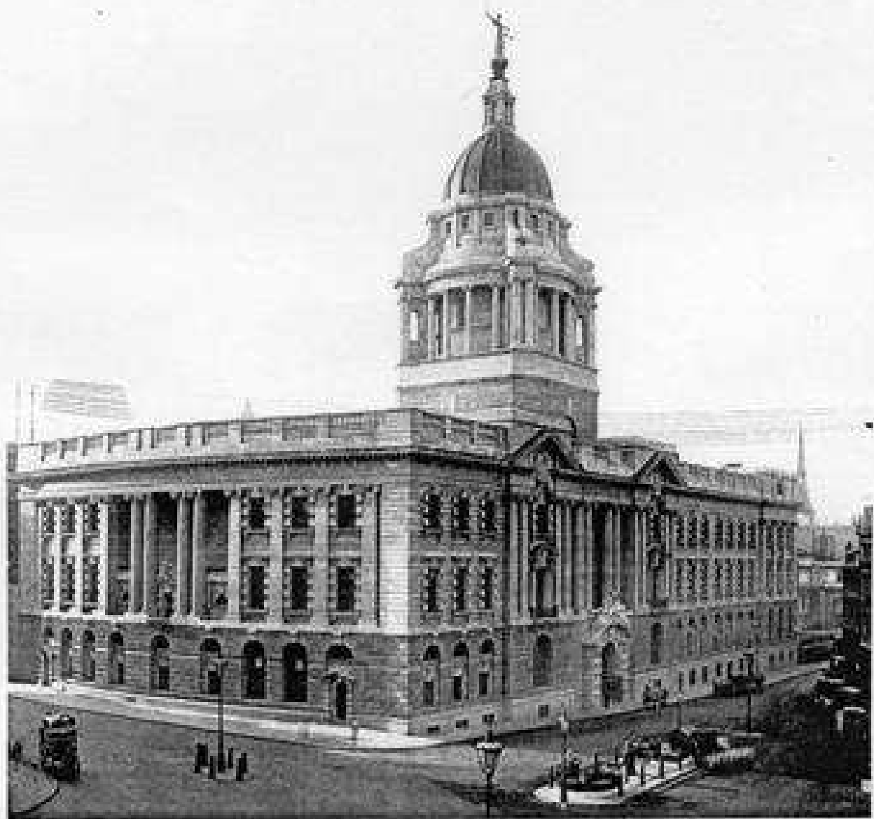
THE NEW SESSIONS HOUSE, OLD BAILEY, E.C. — ARCHITECT: THOMAS S. W. BOUNTFORD. Solid bronze casements throughout, supplied by The Crittall Manufacturing Co. Ltd.
