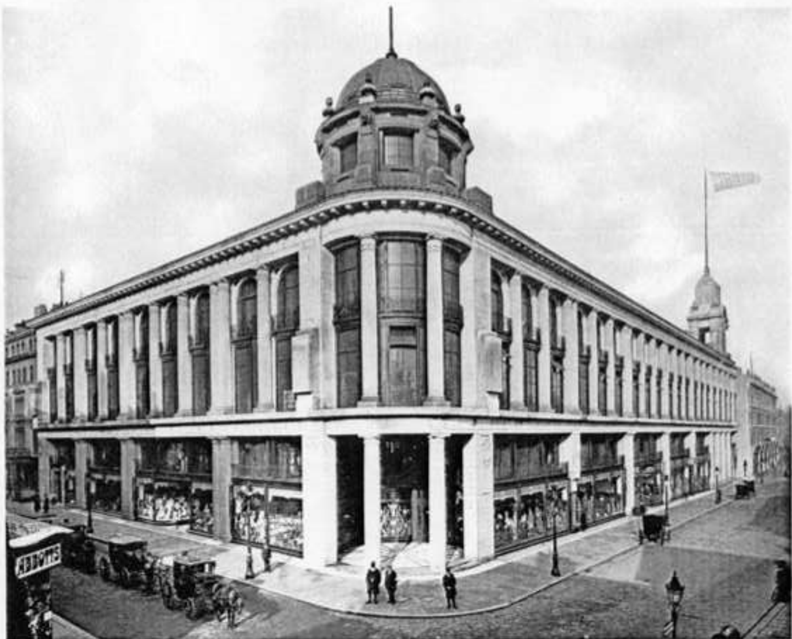
MESSE S . WILLIAM WHITELEY'S STORES, BAYSWATER, LONDON. Architects: JOHN BELCHER, R.A. and J. JOASS. General elevation showing large openings completely filled with Crittall Solid Steel Casements with ornamental mullions and transoms. All the windows and mullions on the first floor are treated with our special Koperoid Process.
